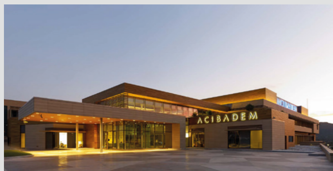
Ortakent Mah Gölbaşı Sok No:11, Bodrum 2015 Progettista / architect : Lina Mimarlik - Istanbul Norm Architects - Istanbul
