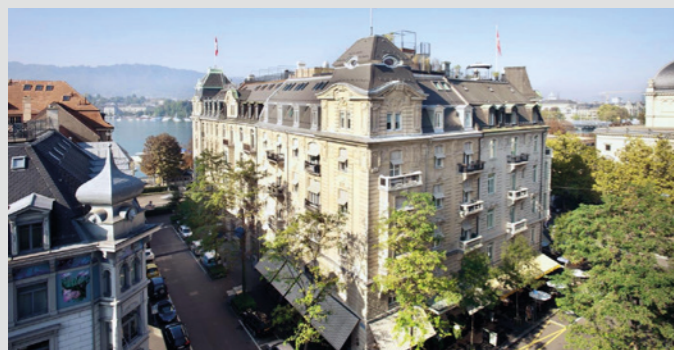
Dufourstrasse 4, Zurich 2012 Progettista / architect : Miller & Maranta - Basel IDA14 by Karsten Schmidt - Zurich
